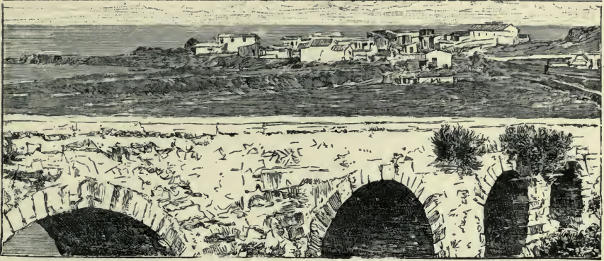
Roman Bridge at Porto Torres.
